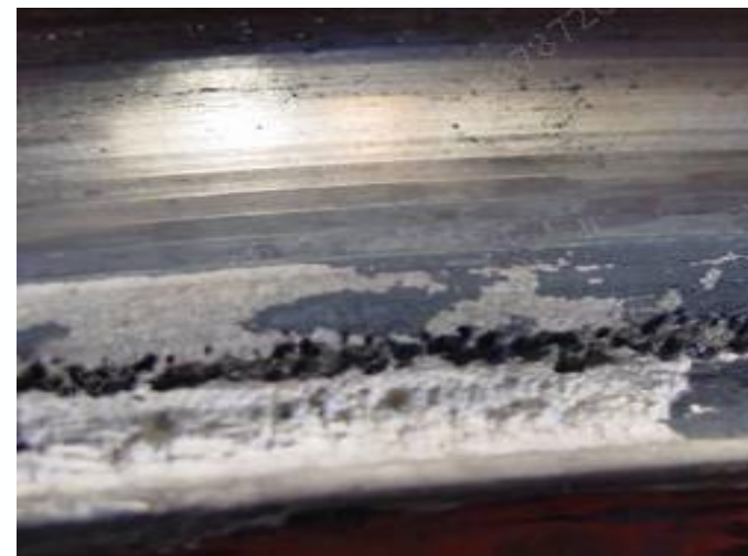
Example of carbamate corrosion
