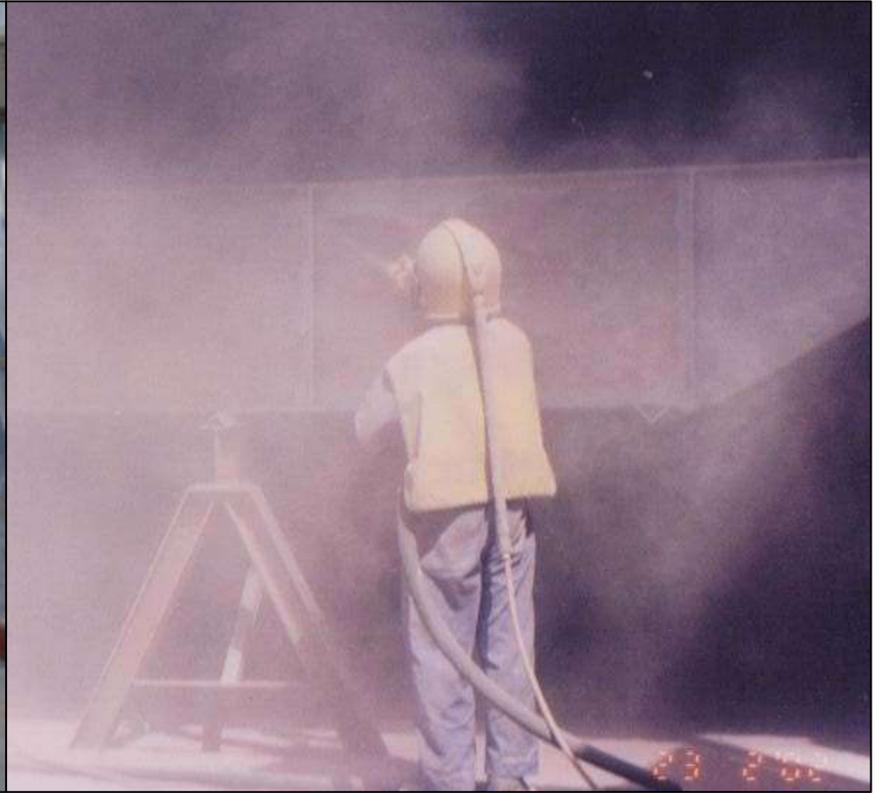
Encapsulated Abrasive Media blasting can reduce dust levels as much as 98% compared to conventional abrasive blasting
