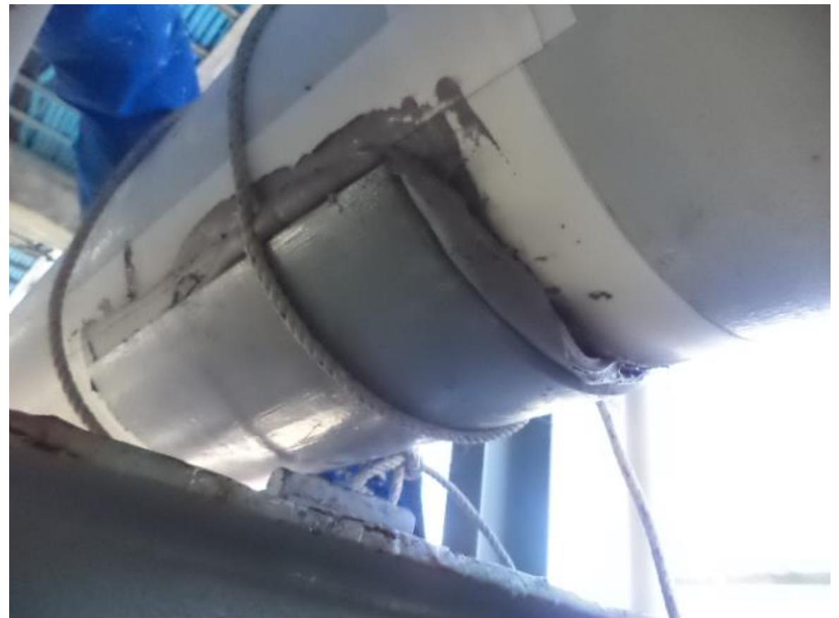
Bond metal plate with corroded pipe
