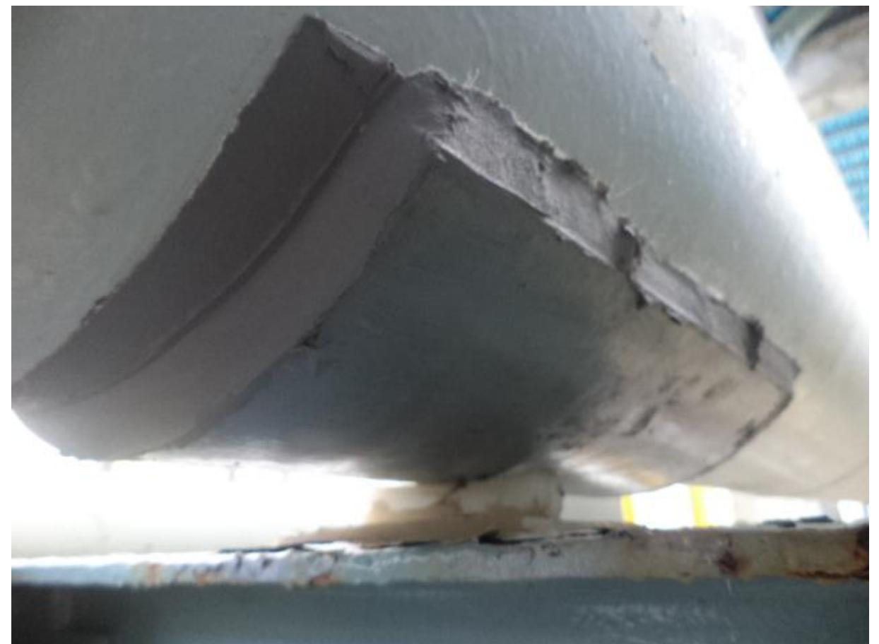
Bond metal plate with corroded pipe
