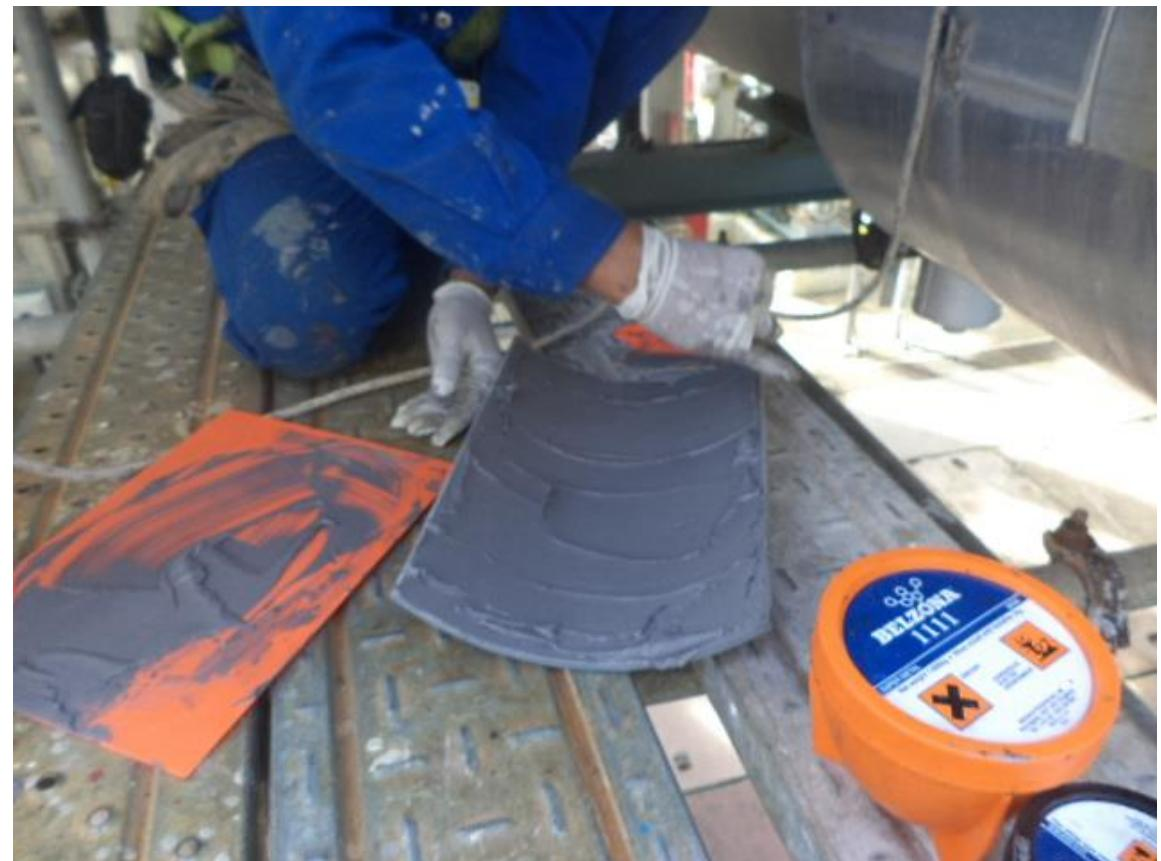
Apply Belzona 1111 on the metal plate
