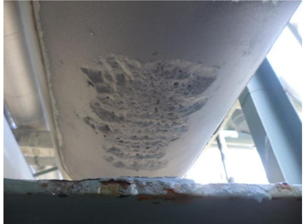
Condition of Corrosion Under Support – After Wet Blasting
