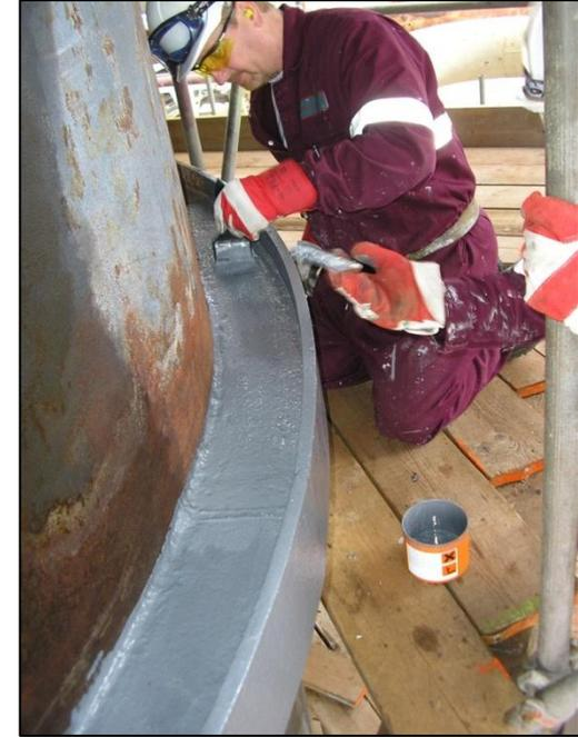
Application of Heat Activated Coating System to Manually Prepared Surfaces
