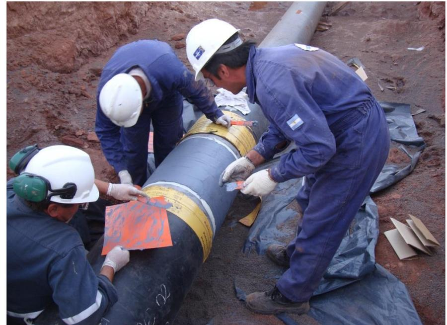
Further Layers of Composite Resins and Reinforcement Fibres applied to Complete the Application.
