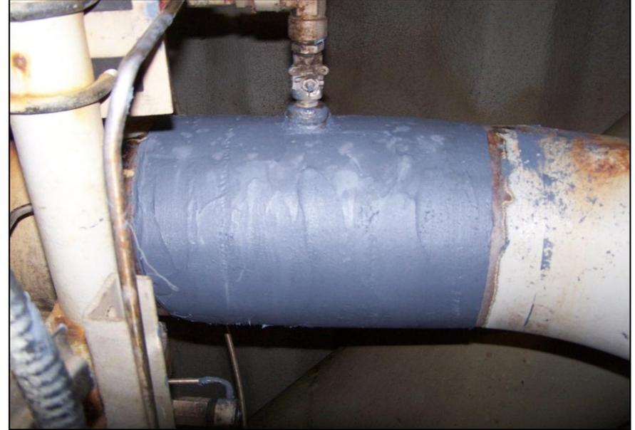
Repair to various produced water lines suffering localised wall thickness loss and through wall defects operating at a pressure of 80 bar. Composite repair applied at 14mm thickness and 6 layers of composite reinforcement
