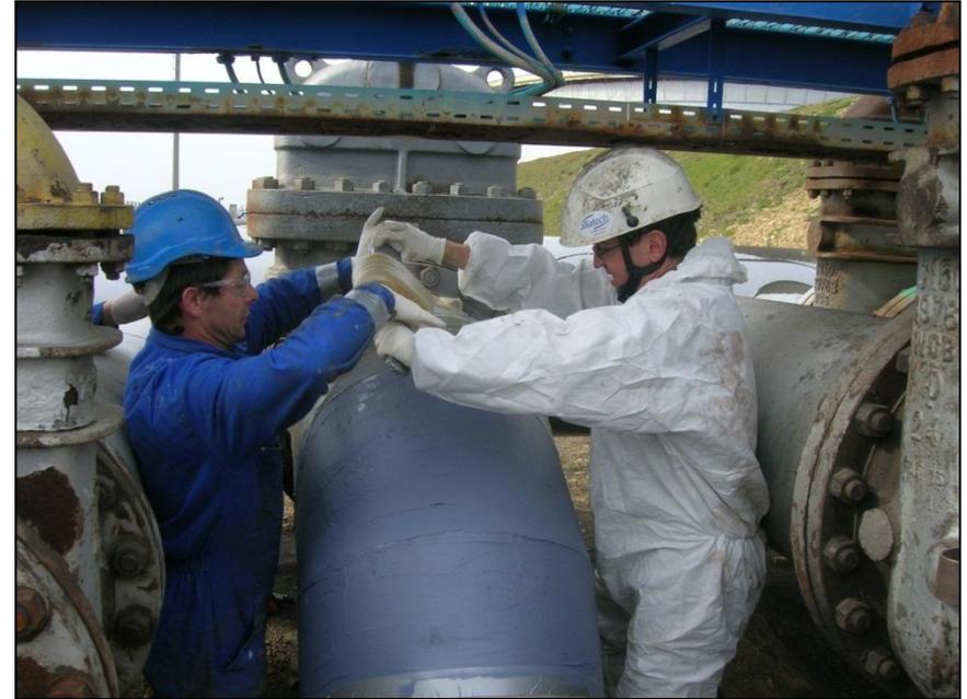
Repair to 34" Crude Oil Line suffering localised wall thickness loss from 6.2mm to 2mm operating at a pressure of 19 bar. Composite repair applied at 5mm thickness and 4 layers of composite reinforcement
