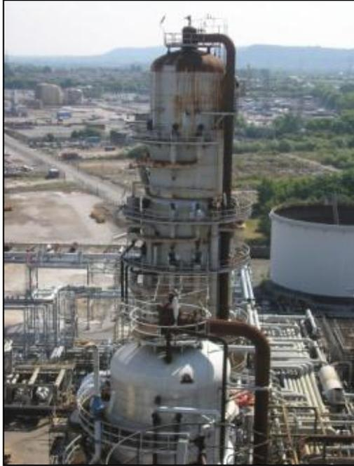
Severe CUI on distillation columns and fractionator towers operating between 50-120°C
