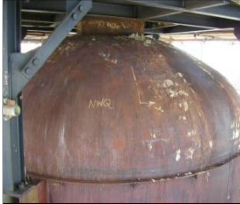
Manual preparation of the steel substrate using scrapers and wire brushes
