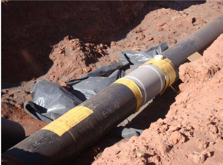
Application of Base Layer of Composite to Repair Pitting
