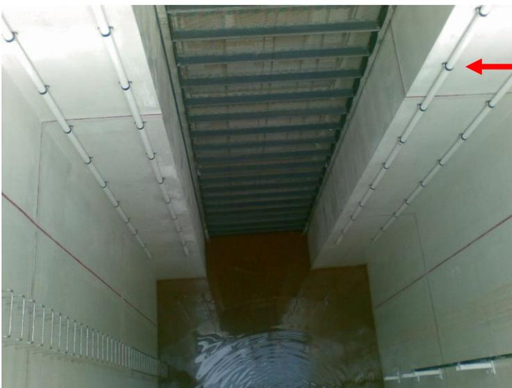
Retractable anodes housed within PVC pipes
