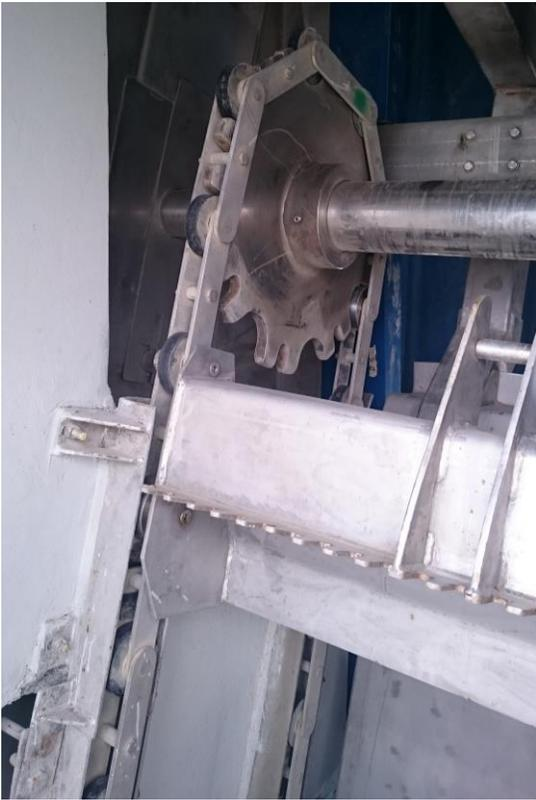
**Figure 7: Continuous Chain Raked Bar Screen**
