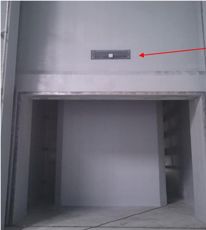
**Figure 2: Installed Strip Anode**
