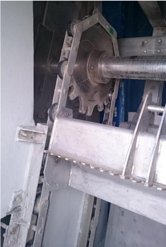
**Figure 7: Continuous Chain Raked Bar Screen**
