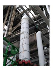
No requirement for scaffold/insulation strip, radiography of 2 x supports, UT of 10 welds
