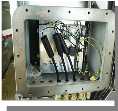
An M2 sensor fitted with armouring to the cable and a hazardous area gland
