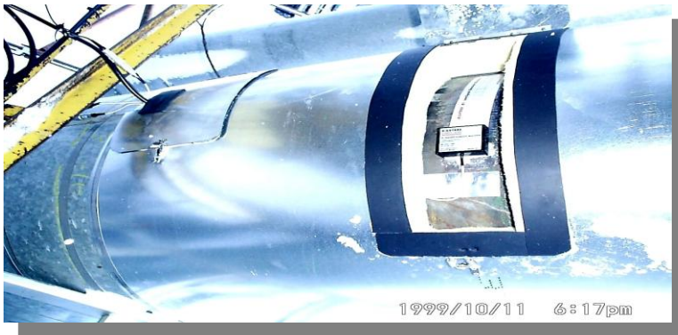
M2 sensors Fitted on Pipelines prior to insulation being reinstated
