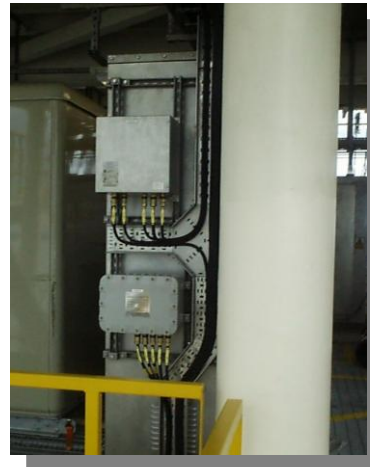
The large hazardous area enclosure containing a fixed DL1, multiplexer and a single board computer that provides data collection, control and data transfer via the BP Ethernet Network on the unmanned HOTON platform in the Southern North Sea
