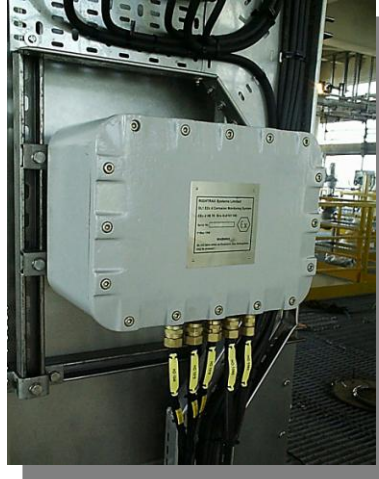
The large hazardous area enclosure containing a fixed DL1, multiplexer and a single board computer that provides data collection, control and data transfer via the BP Ethernet Network on the unmanned HOTON platform in the Southern North Sea
