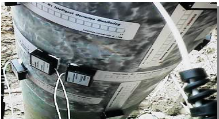
Multiple M2 Sensors fitted to subterranean Pipeline Prior to coating reinstatement and back filling
