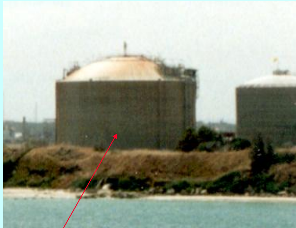
Concrete Bund Wall, inner steel tank.
